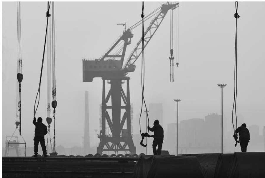
SALON HM - Yi Wu, China, Construction Site
